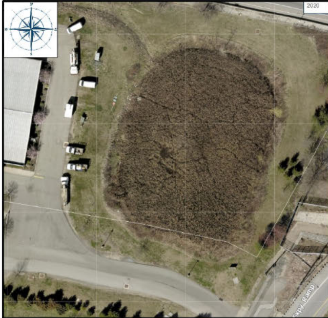
2020 – Stormwater retention basin. (1)
